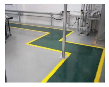
Reground and bio-based plastic materials can also be used within the PVC mix that doesn't compromise the robustness or durability of the tiles' performance. Additionally, when the flooring reaches the end of its lifespan, the tiles are fully recyclable.
